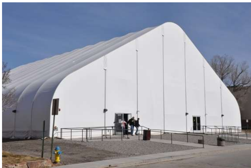
Figure 3 Alternative 1 - Pre-engineered Fabric Structure
