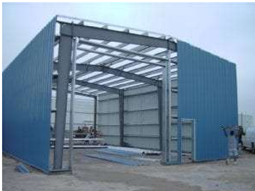
Figure 4 Alternative 2 - Pre-engineered Steel Structure
