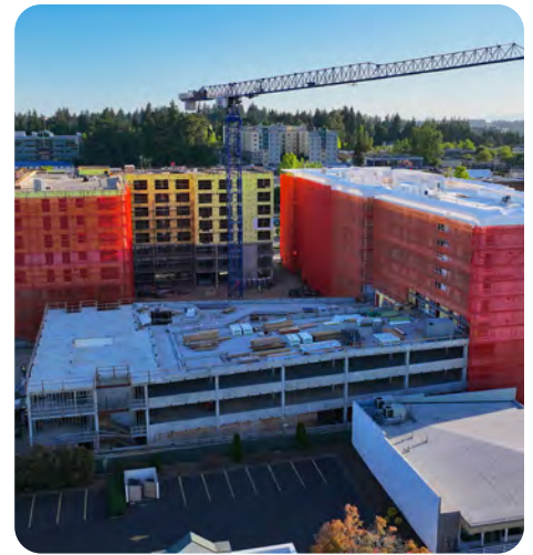
ABOVE: Construction of Ember Apartments Circa 2023
