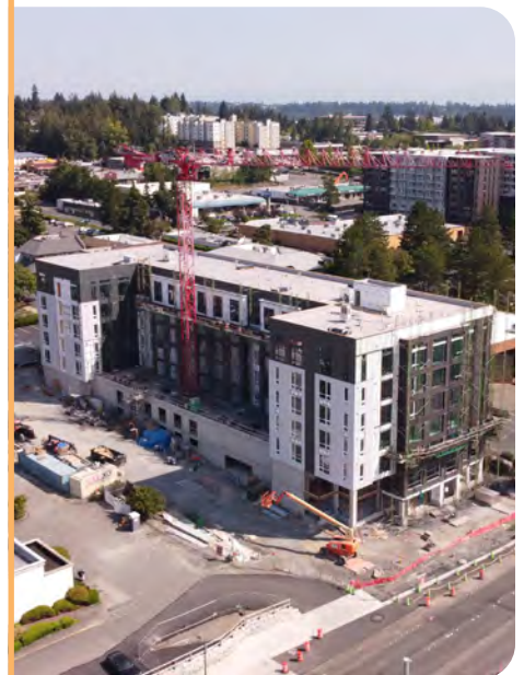
Construction of Koz on Alderwood Mall Boulevard
