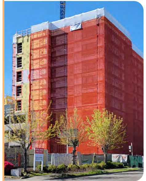
Ember Apartments under construction circa 2023
