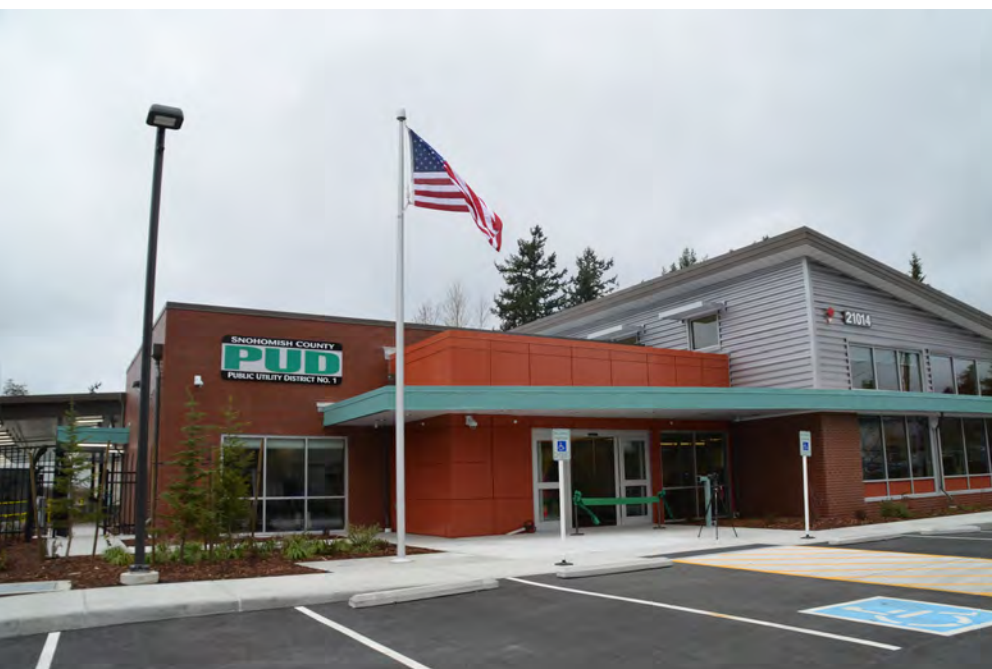
SnoPUD Office in Lynnwood
