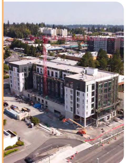
Construction of Koz on Alderwood Mall Boulevard
