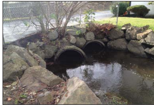
Looking downstream to inlet of Casa del Rey Culverts.
