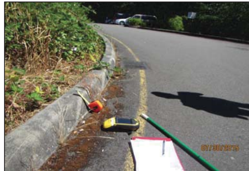
Curb within Eunia Plaza parking lot that berm could tie in to.
