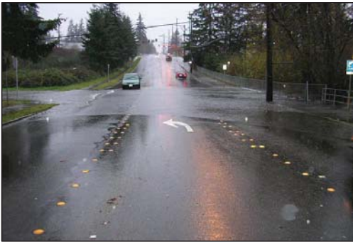
December 4, 2007 overtopping of 188th Street SW.
