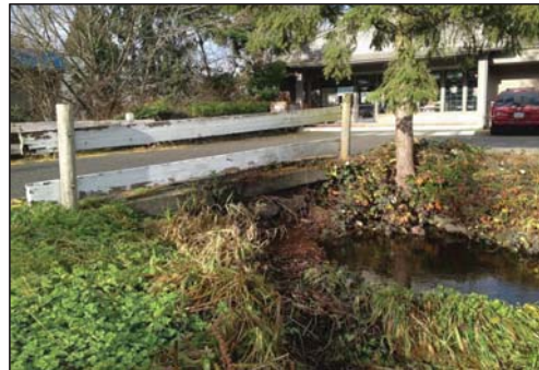
Looking upstream to existing driveway culvert crossing for Parkview Plaza.
