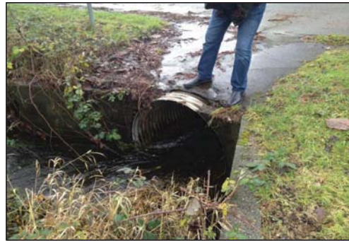
Looking downstream to existing culvert inlet at 191st ST SW.
