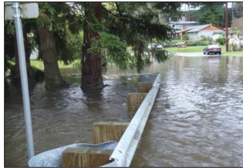
November 23, 2011 flooding of 190th St SW, looking west.
