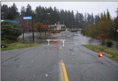
December 4, 2007, Flooding of Old 196th looking east
