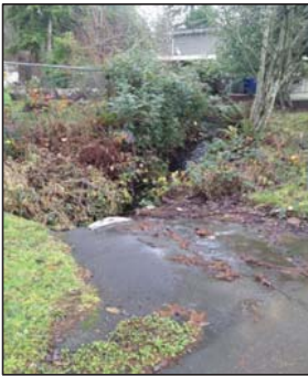
Looking upstream to existing channel and culvert inlet at 191st ST SW.
