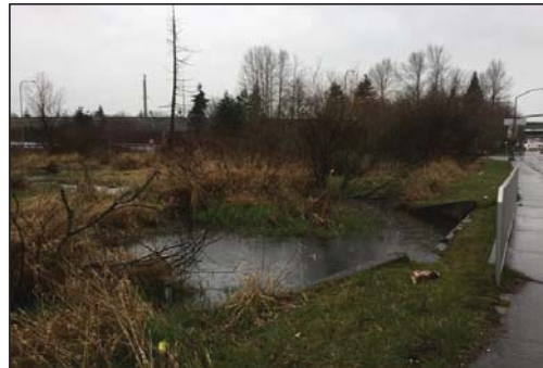
Inlet of Scriber Creek culvert under 44th Avenue W.
