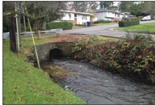
Looking upstream to outlet of existing 189th St SW culvert.
