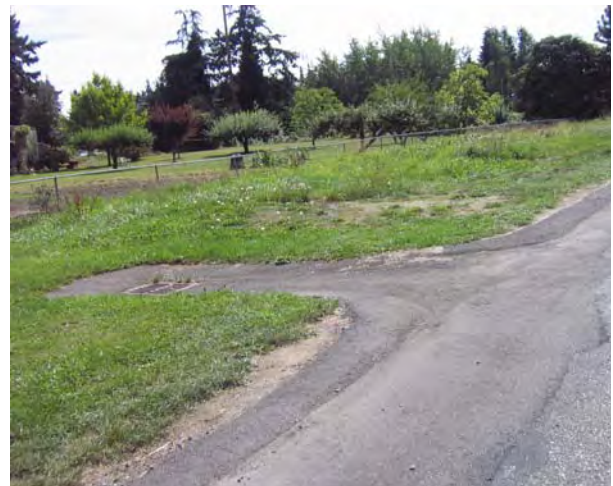
Figure 4. Wide road shoulders in the Hall Lake basin are ideal for street edge treatment swale retrofits.
