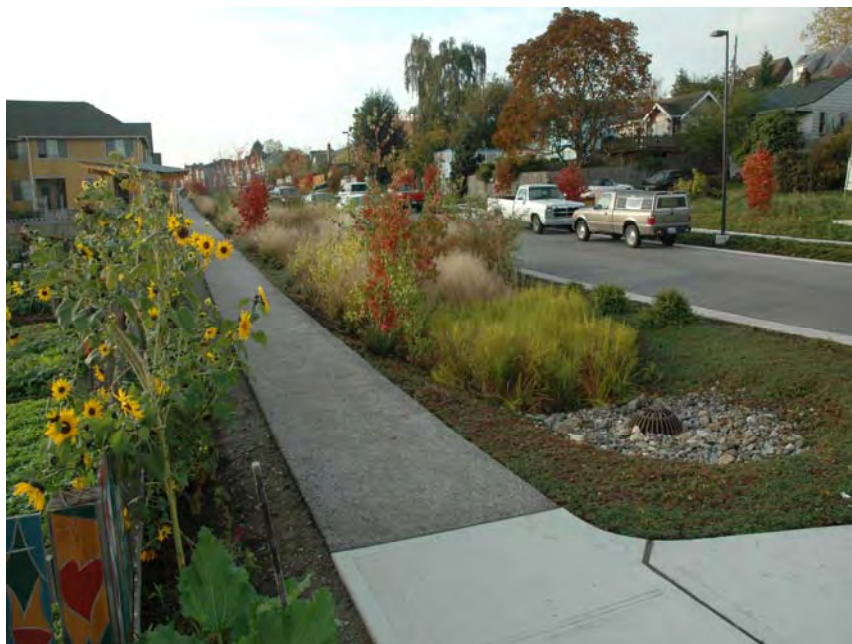
Figure 4-3. Bioretention swales used for flow control and water quality treatment of roadway runoff.
