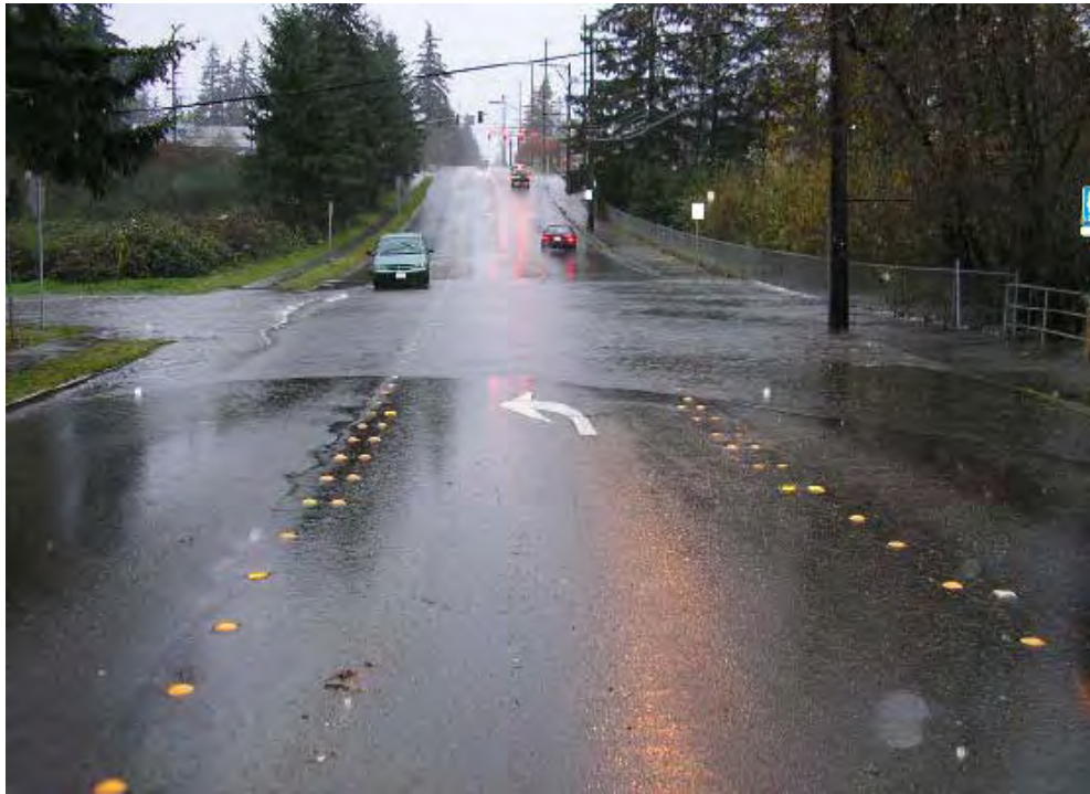
Figure D-1. December 3, 2007 flooding of Scriber Creek at 188th Street SW.
