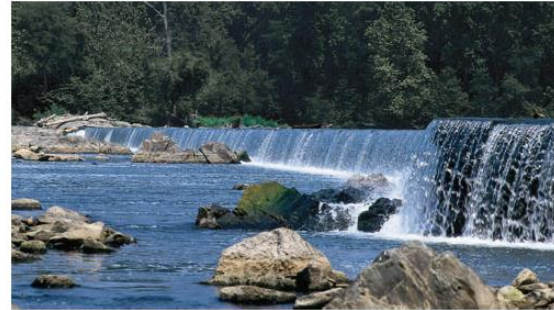
Fig. 2-16 Stay away from dams. The chances of surviving an aquatic emergency involving a dam are slim.
