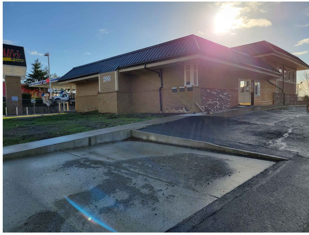
NORTH WEST CORNER
