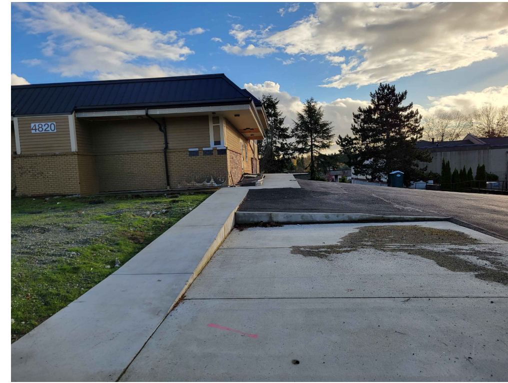
NORTH ELEVATION LOOKING SOUTH
